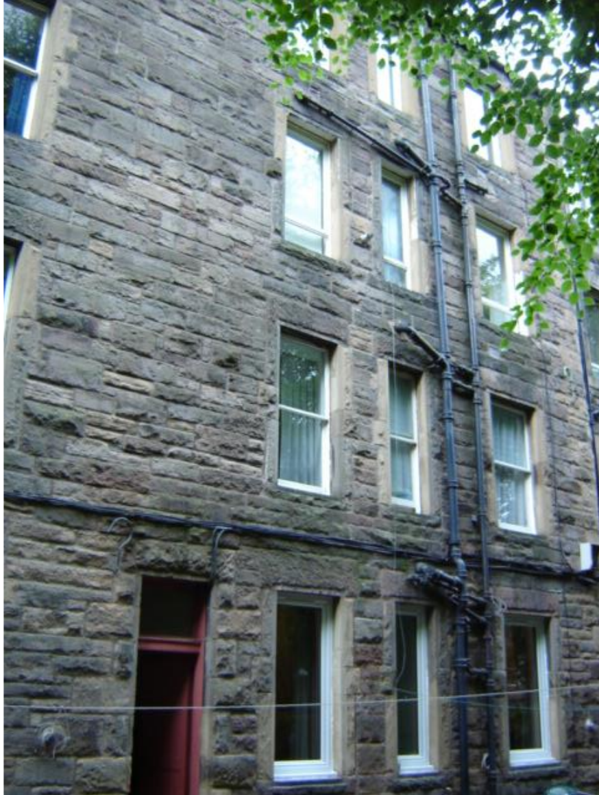
Ground floor 1890s tenement flat with solid stone walls and combi boiler
